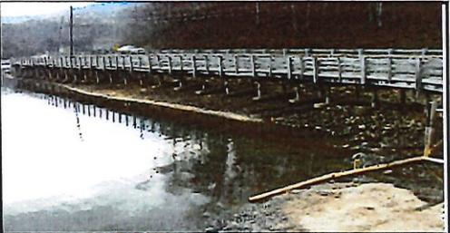
**Justification:** Current boardwalk is becoming dilapidated and unsafe. Aside from wood rot and weathering the footings are becoming unstable due to scour and pose a danger of collapsing. Boardwalk is part of the Town Center Master Plan and is an important means of moving people between the Town Center and Morse Park. An enhanced boardwalk would be safer and further enhance the aesthetic of the Marina. This project also is identified in the Comprehensive Plan as a priority.
