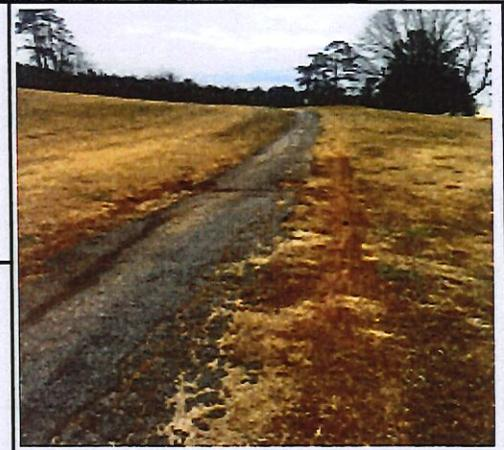
**Justification:** The existing cart path system has been degrading for a number of years. The existing paths are too narrow to support golf carts and maintenance equipment creating a safety hazard. Many edges have crumbled due to inadequate sub-base preparation before installation.
